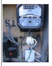
As time goes by, products are being released onto the market at moderate prices to carry out some or all of these functions. See for example the Electrisave, sensor pictured above. The top part of the unit, (white clip on a grey wire), is a 'current transformer' sensor. This clips over an incoming cable and senses the current in the wire magnetically without requiring an electrical connection to be made.
