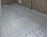
Hilton Scouts and Guides building, underfloor heating pipe laid on insulating base prior to pouring concrete floor. Pipes at optimal spacing for low temperature heat pump operation.
