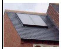
Flat plate solar collector for water heating installed by T4 Sustainability," in roof mounting" (flashed into roof)
